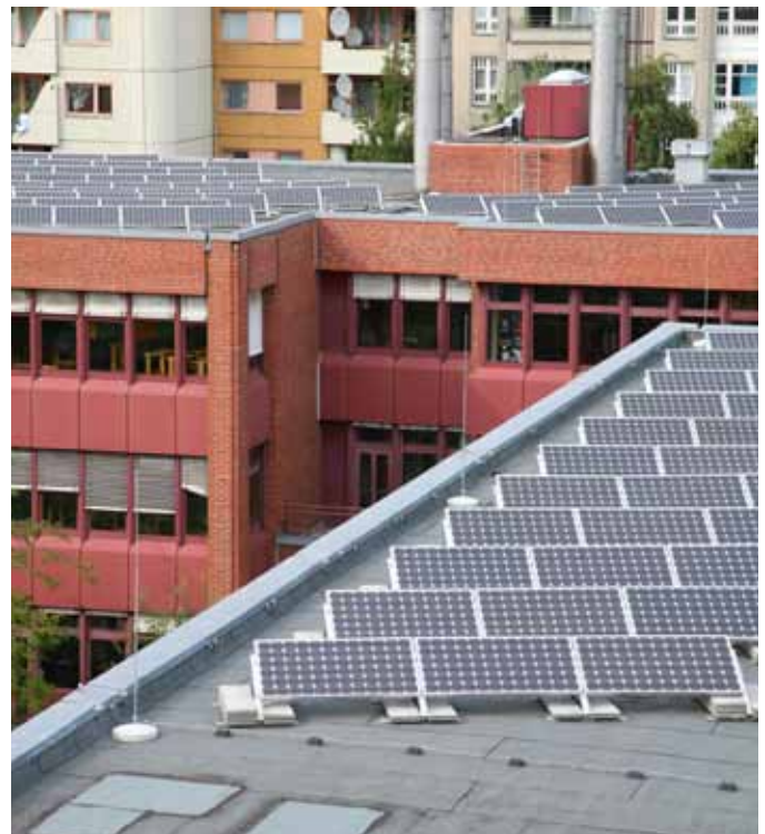
Illustration 9. Large roof-mounted solar array
