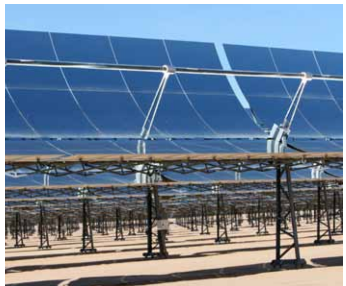
Illustration 3. Parabolic trough solar concentrators
