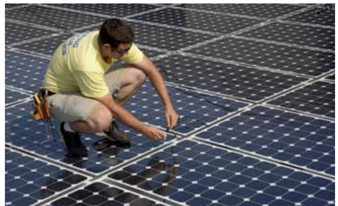
Illustration 8. Man wiring solar panels
